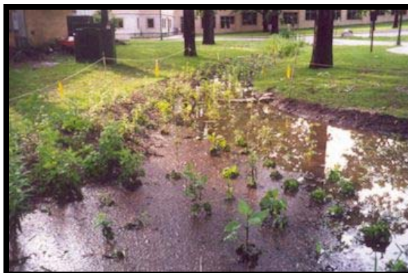
Newly Constructed Bioretention Area
