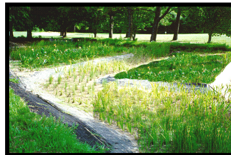
Newly Constructed Shallow Wetland
