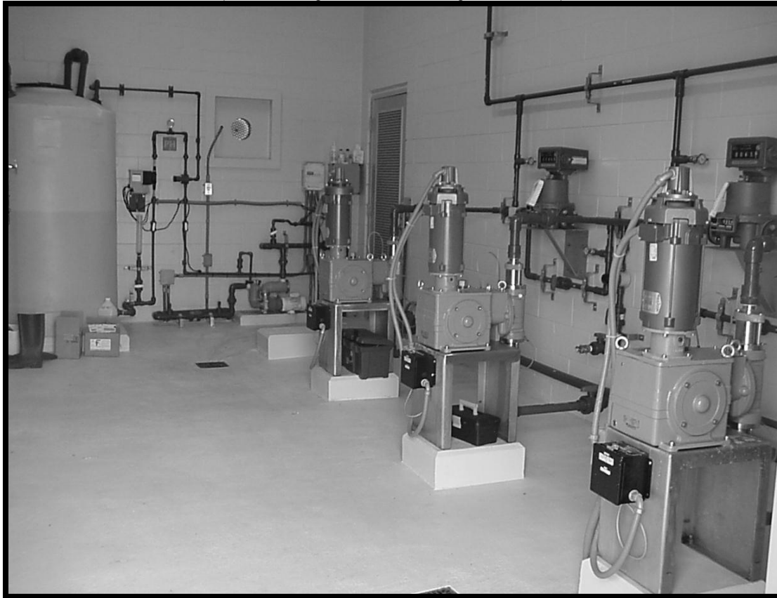
Figure 4-67. Dosing/Injection Components of an Alum Treatment System
