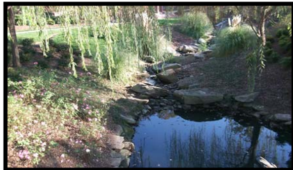
Micropool Extended Detention Pond
