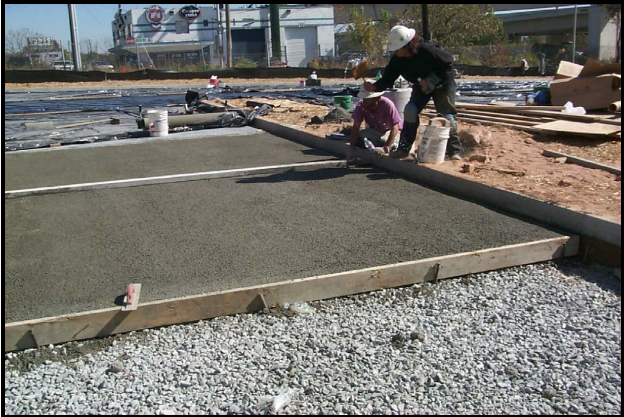
Figure 4-54. Porous Pavement Installation
