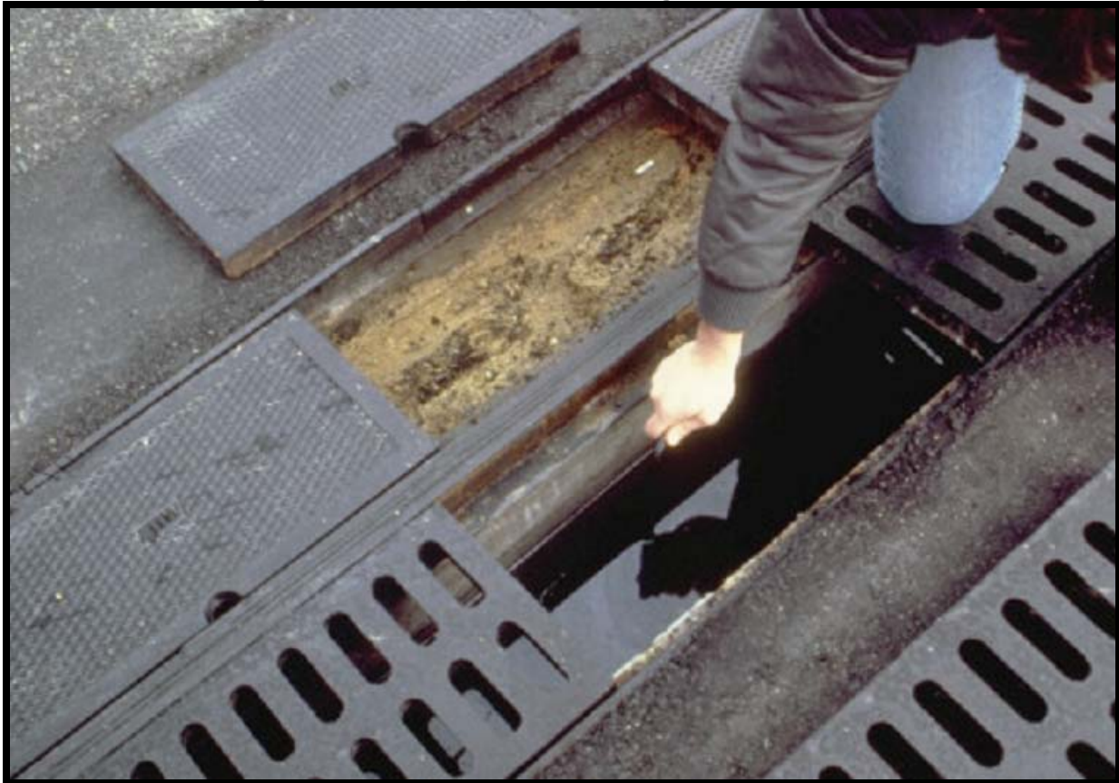
Figure 4-59. Example of an Underground Sand Filter
