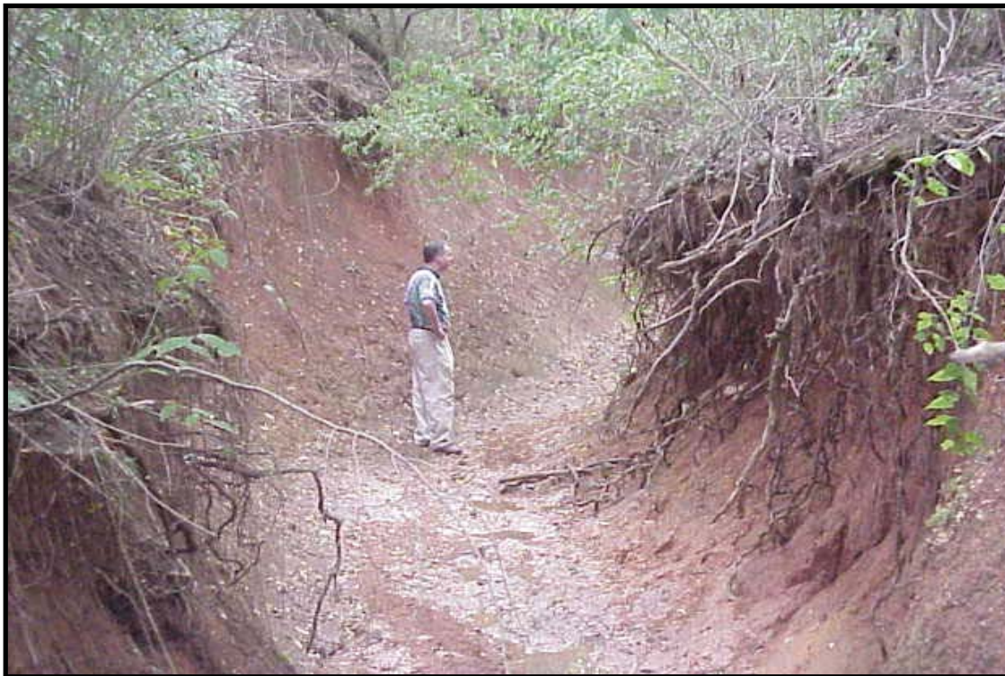
Figure 2-2. Example of Significant Streambank Erosion
