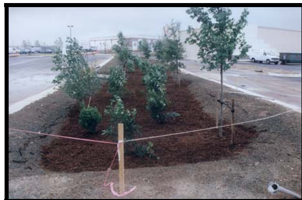
Newly Planted Bioretention Area After Storm Event
