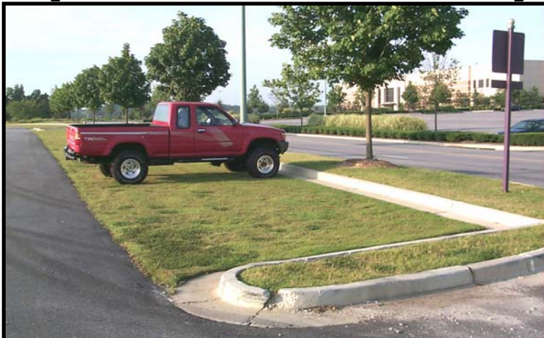
Figure 5-20. Grass Paver Surface Used for Parking
