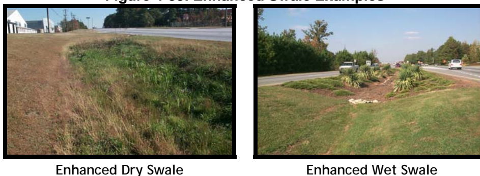
Figure 4-39. Enhanced Swale Examples
