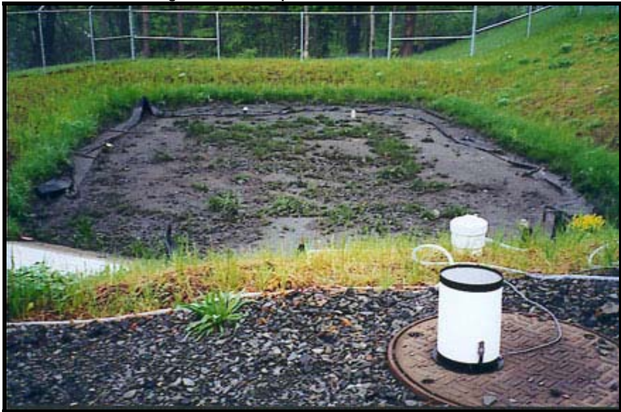
Figure 4-31. Example of a Surface Sand Filter
