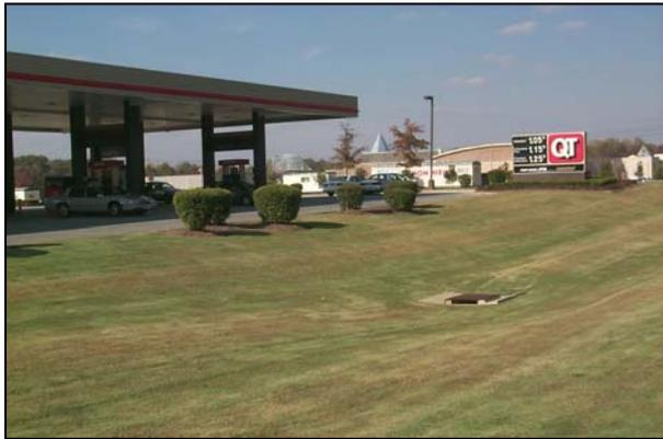
**Description:** Filter strips are uniformly graded and densely vegetated sections of land, engineered and designed to treat runoff and remove pollutants through vegetative filtering and infiltration.
