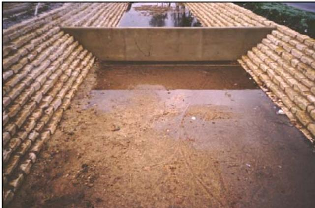
**Description:** Surface sand filters are multi-chamber structures located above ground that are designed to treat stormwater runoff through filtration, using a sediment forebay, a sand bed as its primary filter media and, typically, an underdrain collection system.
